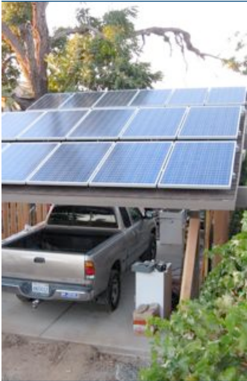
The new solar structure at the Hooper-Rusmore residence doubles as a carport. PHOTO BY NINA RUSMORE
