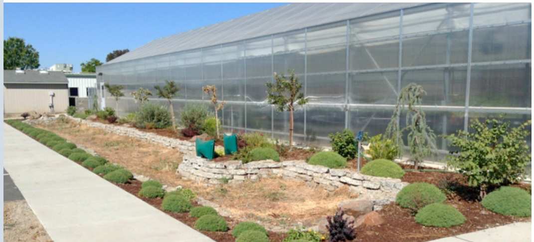
Students recycled concrete walkways to create a retaining wall for the bio-swale. The bio-swale and demonstration landscape are slated for completion in Spring 2014.
